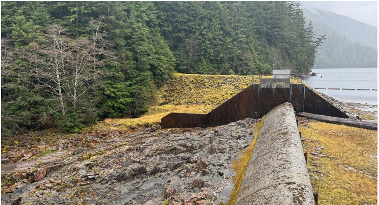
Figure 4-30. Spillway (Photo: Bryant Wright)
