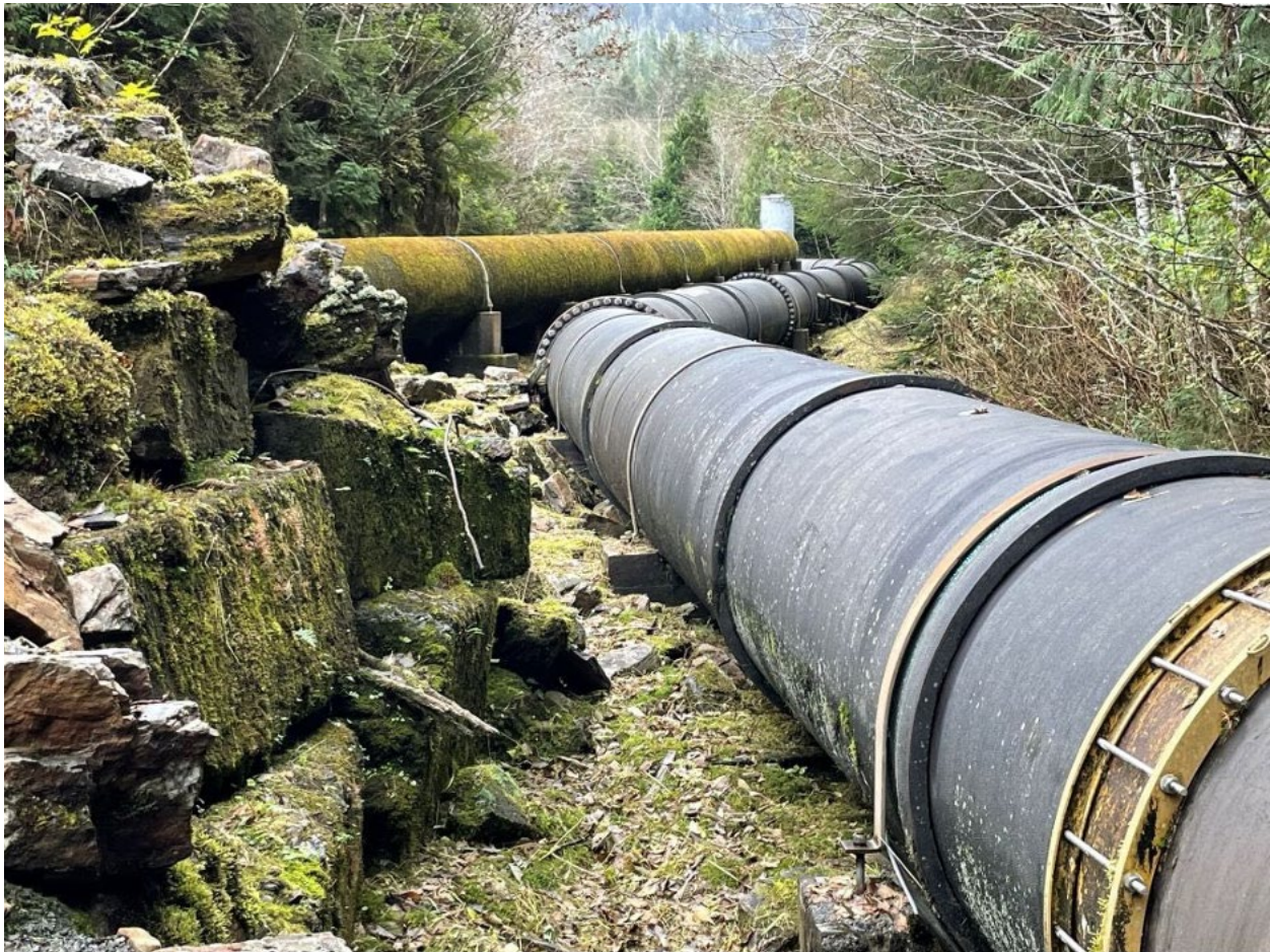
Figure 4-43. Ductile Iron Penstock 2, 2022.
