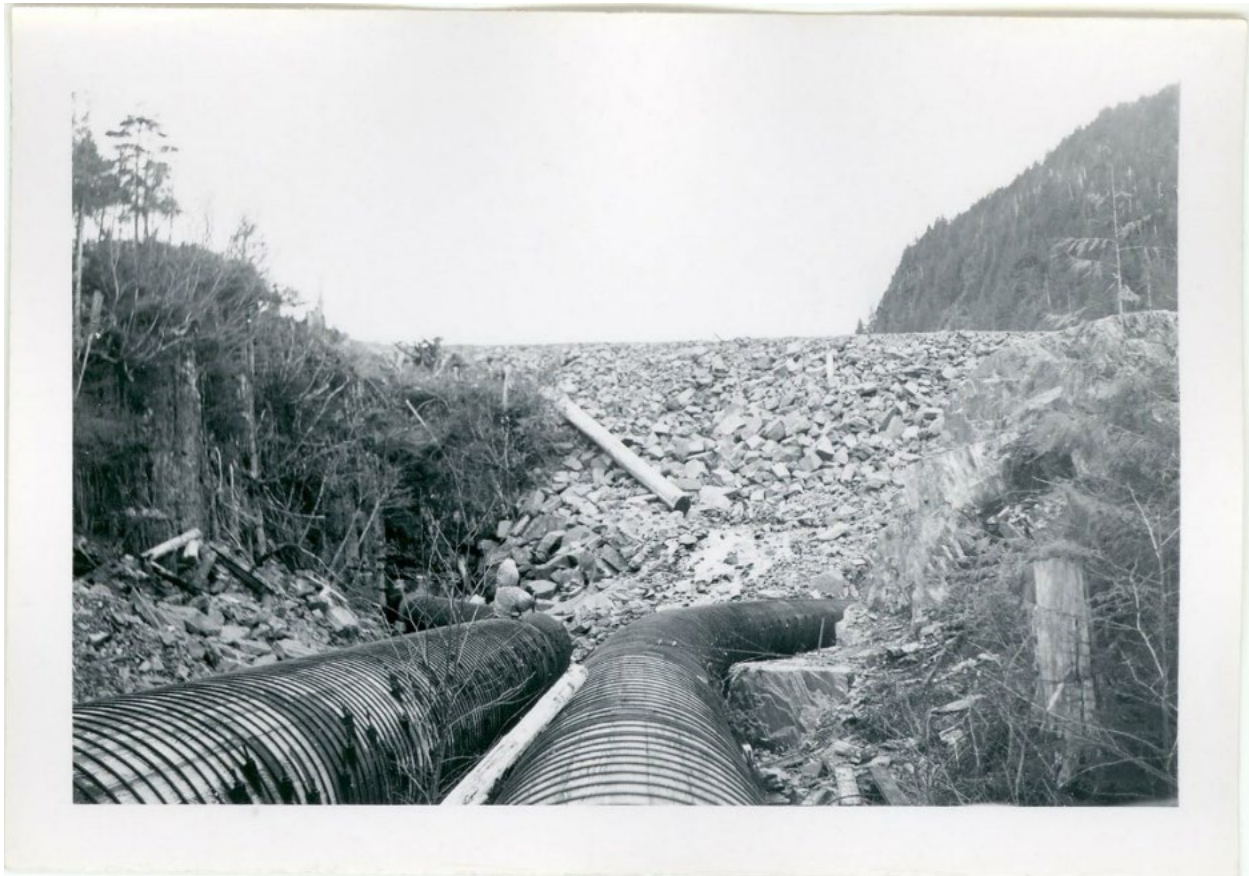
Figure 4-42. Newly Completed Ketchikan Lakes Dam and Penstocks 1 and 2, c. 1958
