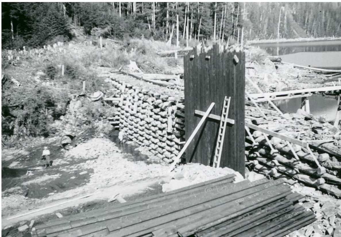
Figure 3-7. Ketchikan Lakes Dam – Core Wall Construction
