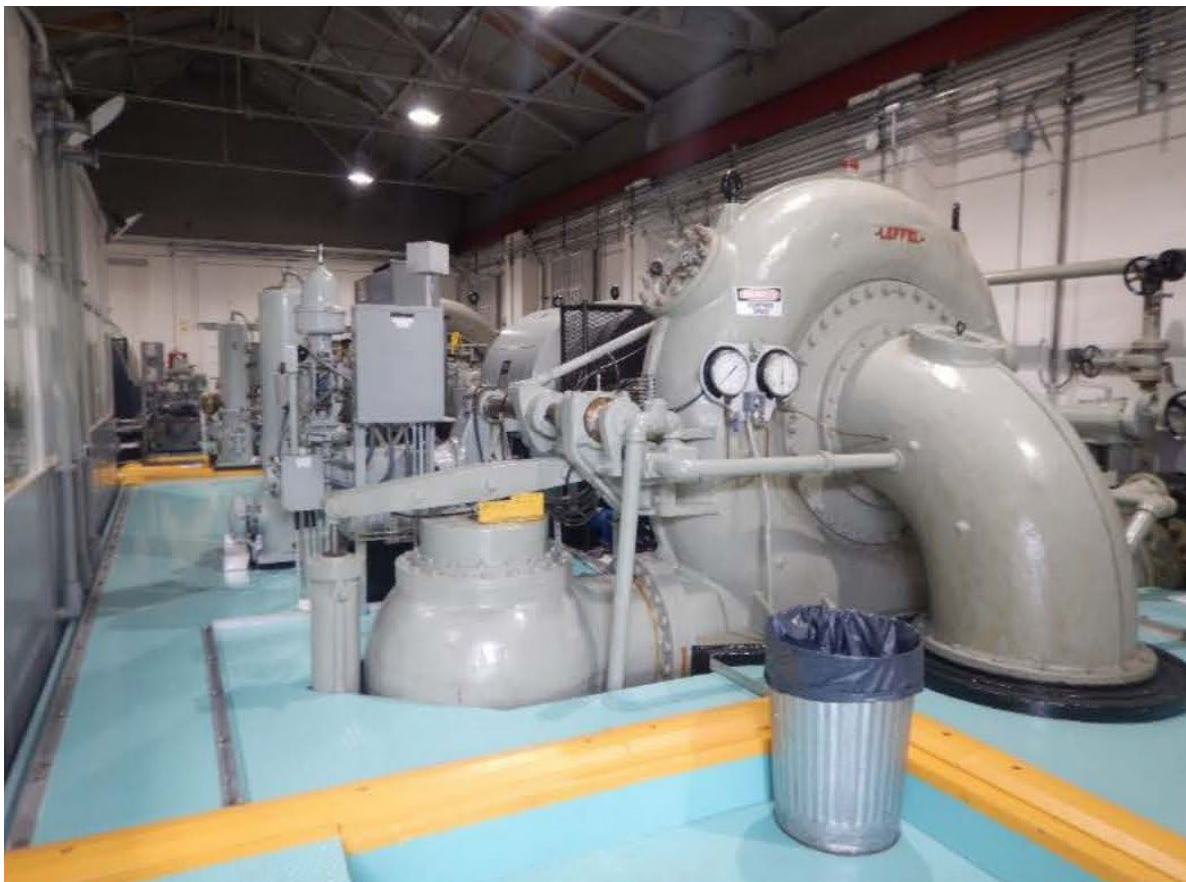
Figure 3-16. Turbine-Generator Units
