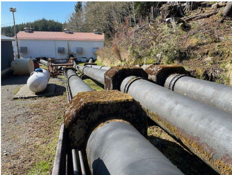
Figure 3-15. Penstocks Entering the Powerhouse
