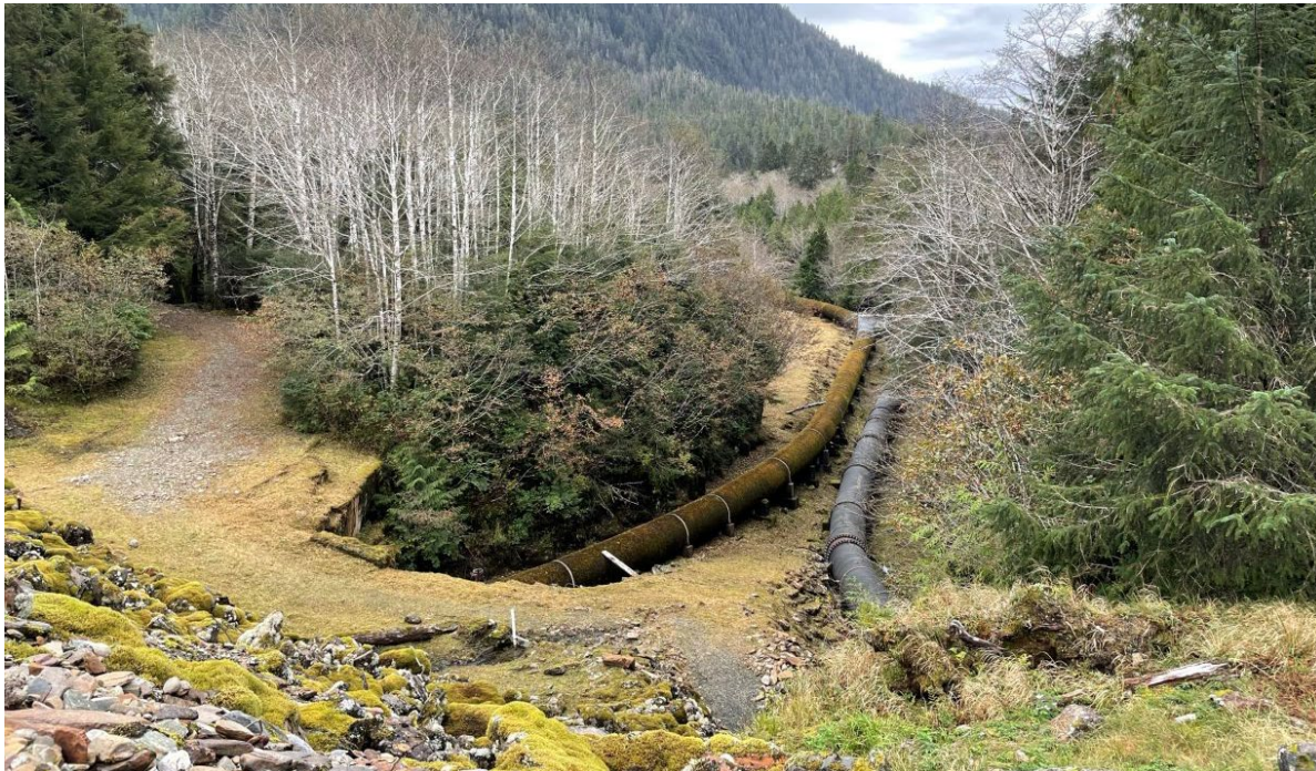
Figure 3-11. Penstocks Downstream of Ketchikan Lakes Dam
