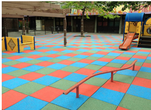
Rubber tile safety surfacing
