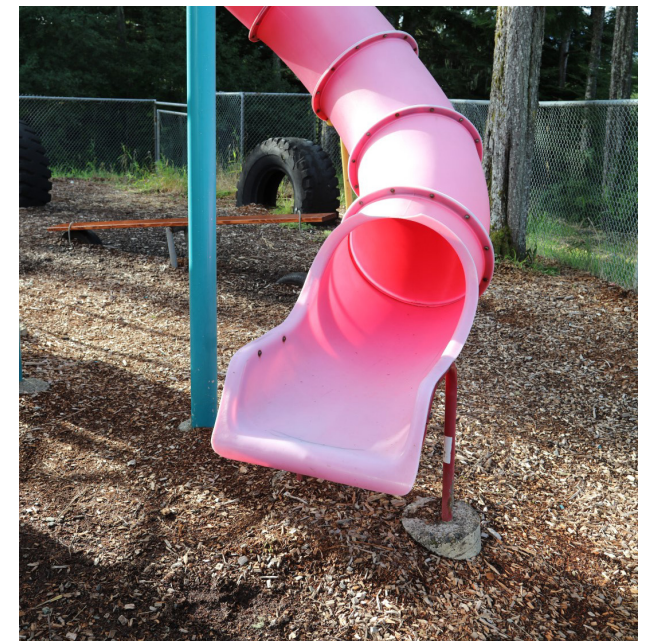
Existing slide with exposed footing
