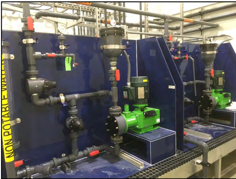
Secondary Chlorination Facility Pump Apparatus
