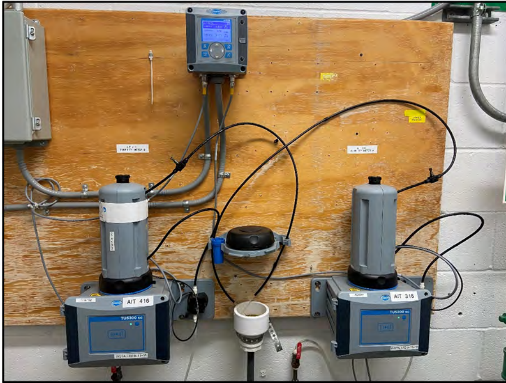
Turbidimeters for Line A and B – Chlorination Facility
