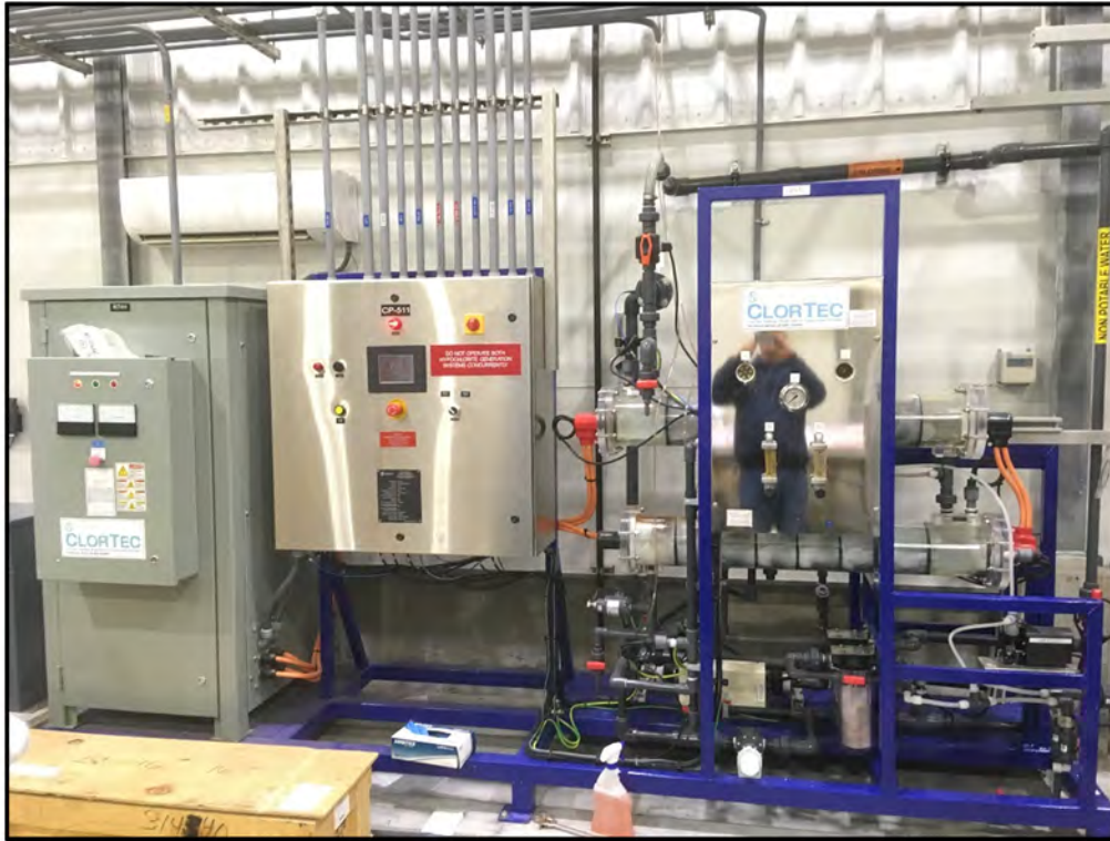
Secondary Chlorination Facility Hypochlorite Generation Systems
