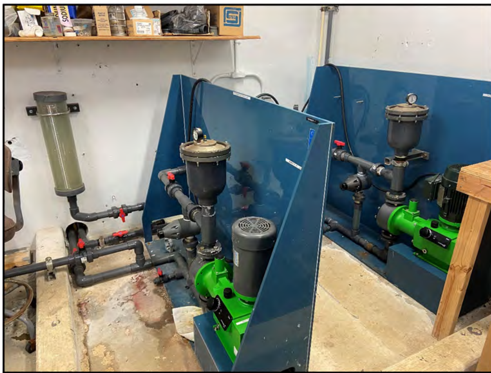
Redundant Hypochlorite Injection Systems - Primary Chlorination Facility
